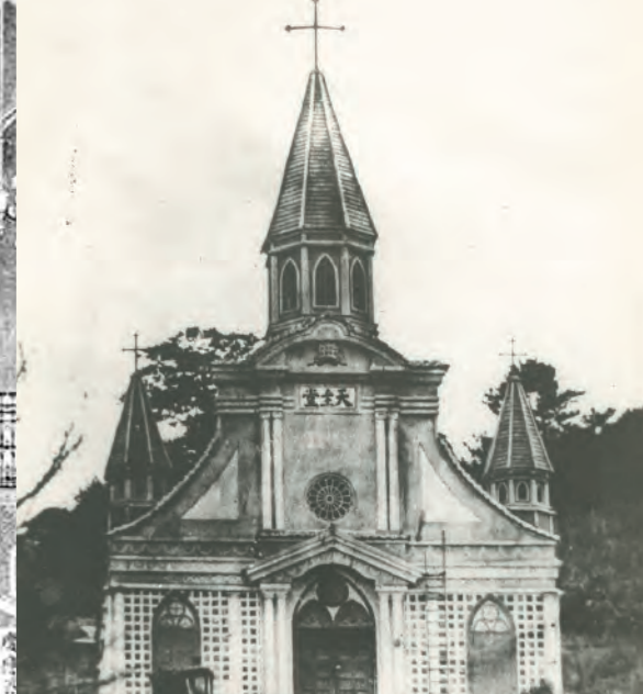
Oura Cathedral (component ⑩) at the time of its construction * Photo reprinted by courtesy of Nagasaki Bunkensha
